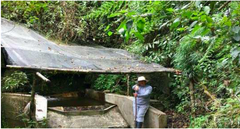
Figure 1: Community aqueduct in Pasto, Colombia (Perugache Salas, 2020).
